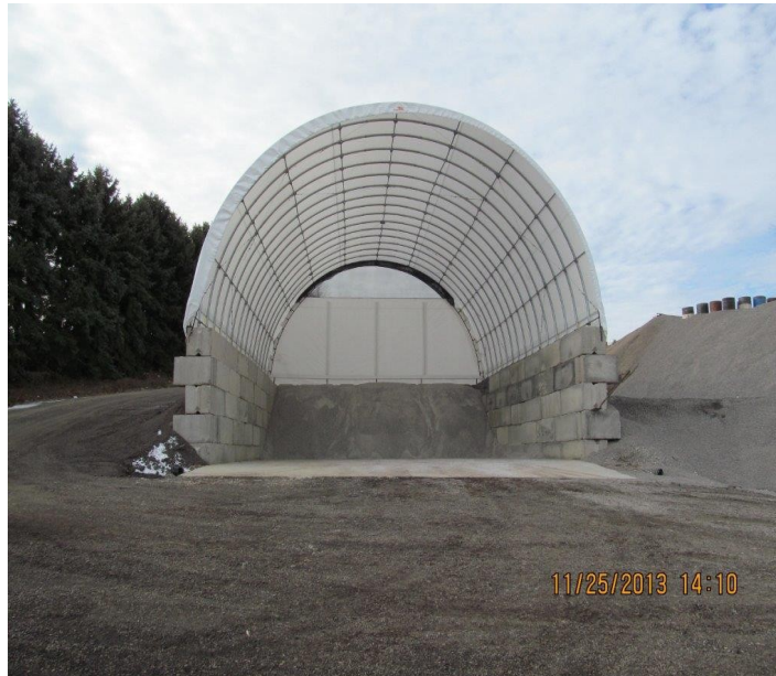
SEWICKLEY TOWNSHIP'S NEW SALT SHED
