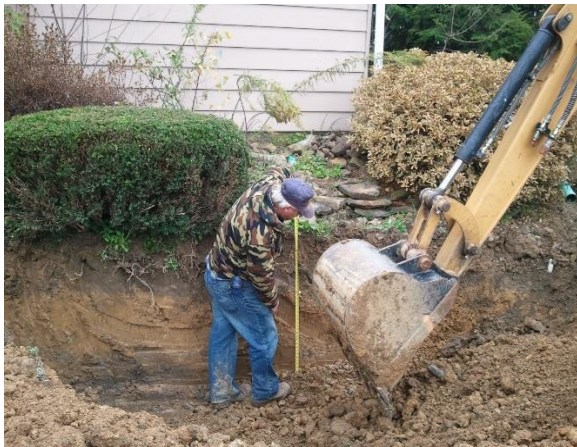
Excavate a drywell at least 10' from foundation
