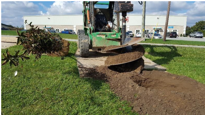
Plywood sheets protect lawn from compaction
