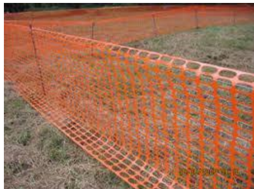
Fencing protects areas from compaction
