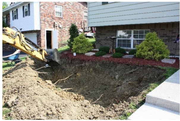
Excavate rain garden at least 10' from foundation
